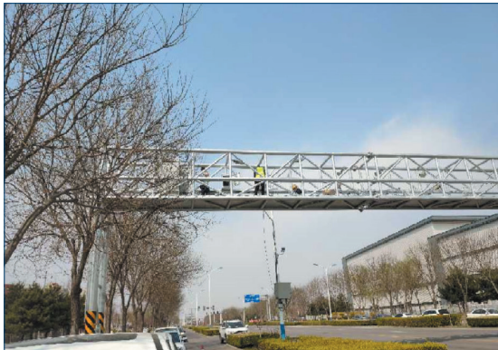
Figure 4. Deployment scenarios of Roadside MEC Equipment (in pole-mounted cabinet).
