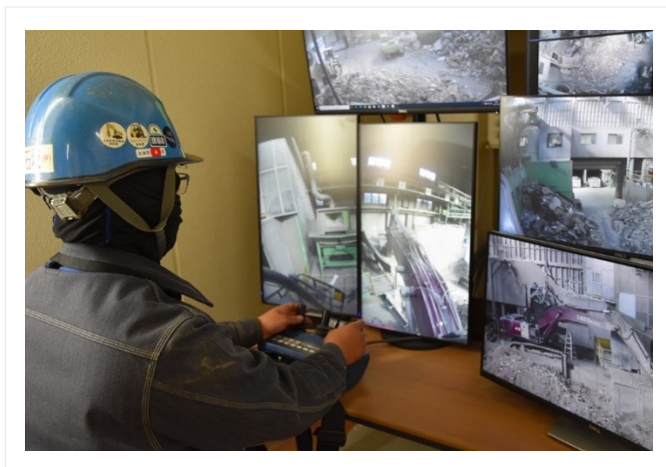
Figure 4. Trained worker remotely controls backhoe over 5G to avoid close contact with hazardous waste.
